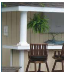
Vinyl Board & Batten Siding on Bar Exterior
